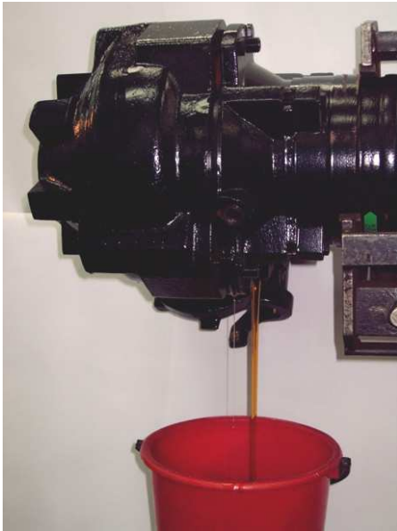
Draining the oil chamber
